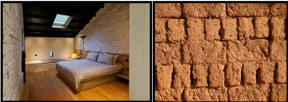
Figure 18: Left. Old building reutilized in modern rural commodity. Right. Local soil wall.
